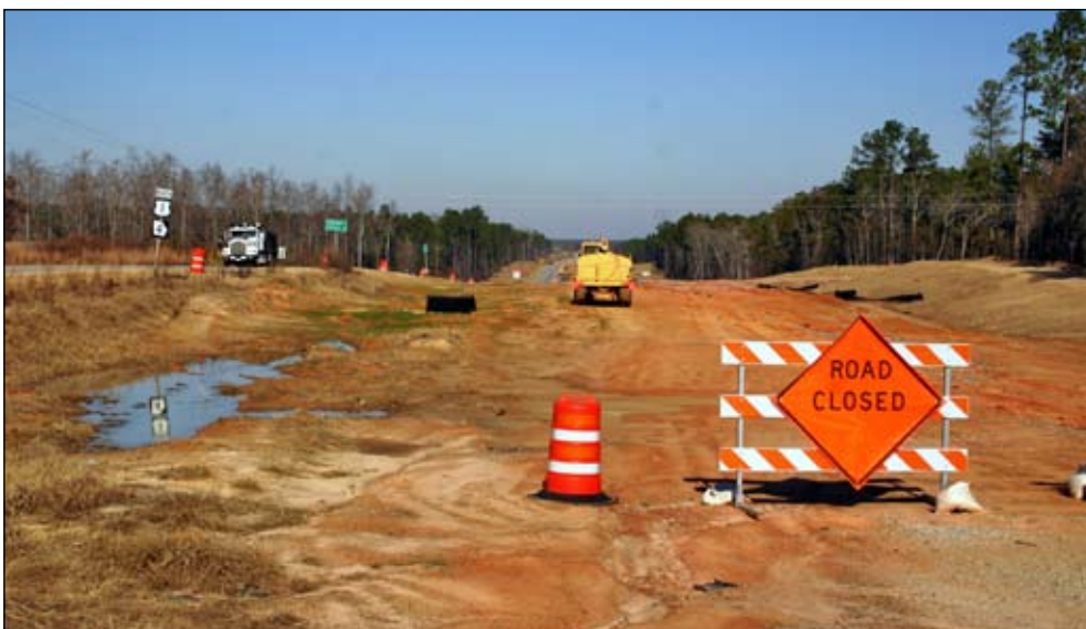
The US 1/SR 4 widening project adds two lanes to a 9.7 mile section of highway.
