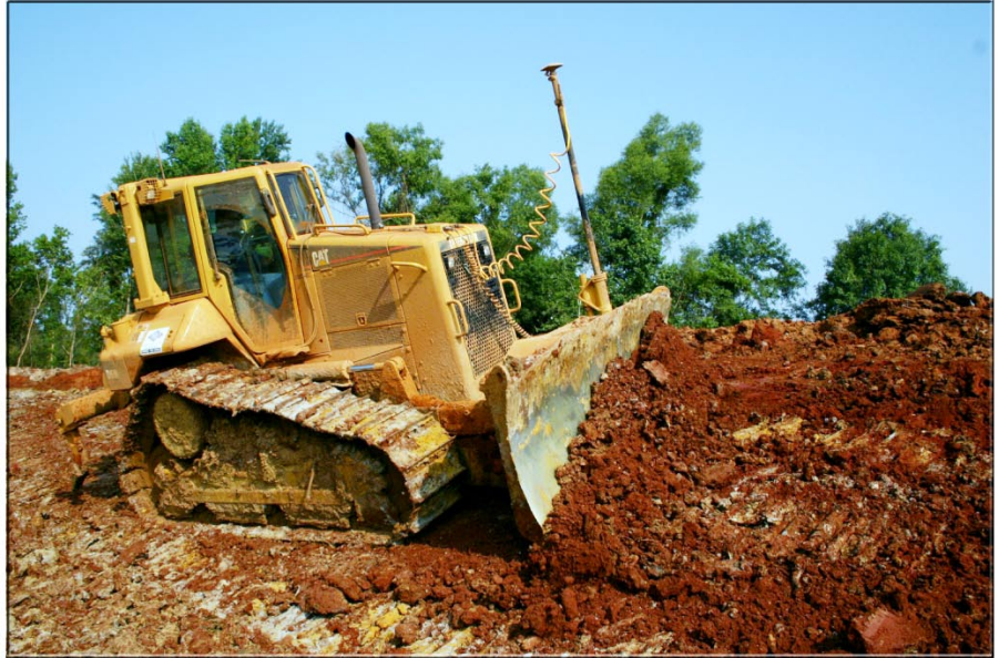
Stanley's Cat D6N w/Topcon's System Five 3D-GPS+ fully automatic machine control
