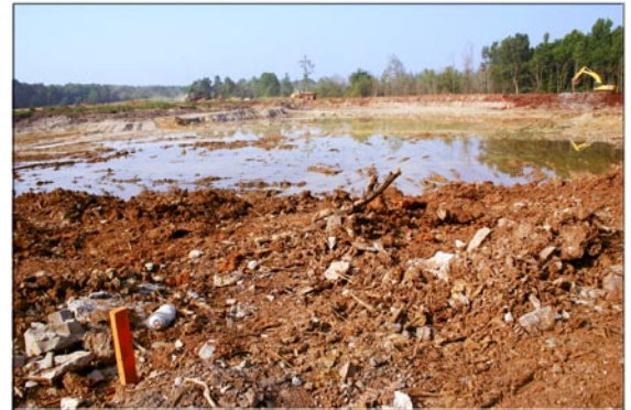
Tough conditions - Heavy clay soils, wetland conditions, and a rainy Spring
