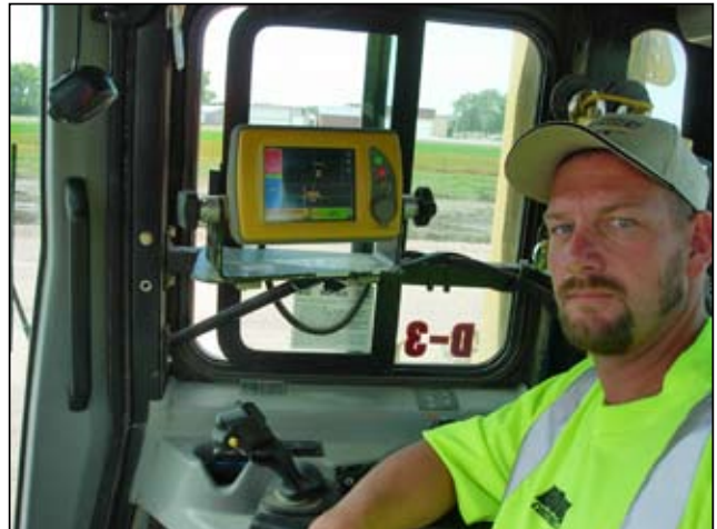
ABOVE: Bowes Construction equipped a second dozer with the Topcon 3D-MC 2 system and a machine control-equipped Caterpillar 140H grader followed closely behind and fine-graded the aggregate. BELOW: The GX-60 monitor shows the precision of the dozer blade positioning for operator LaDuke Palmer.
