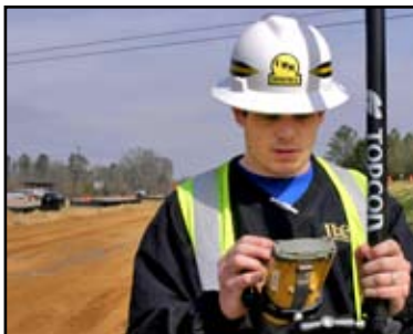
Adam Chance, foreman - GPS fine grading
