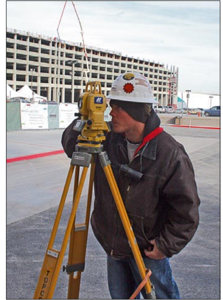
Using a GTS-235W total station simplified the once time-consuming process of establishing control points for Embassy Glass. Field foreman Ché Hecker shot 11 floors in a matter of days using the total station.
