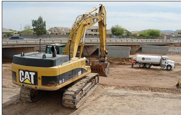
The bridge on Higley Road, a major north-south arterial east of Phoenix, crosses a wash in the Eastern Maricopa Floodway. A lane was to be added in each direction, necessitating the construction of five piers to support each new traffic lane.
