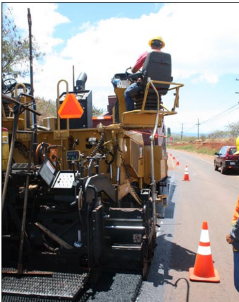
Maui Paving Company using Topcon's Paver System 5.
