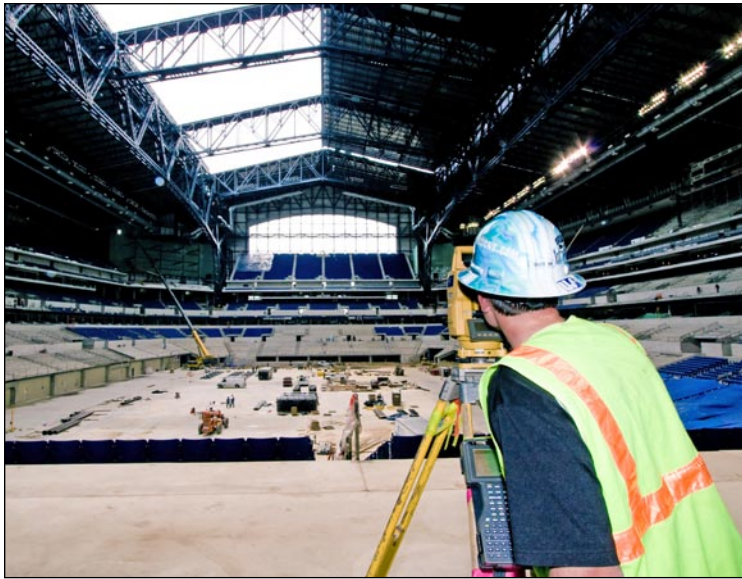
USI Consultants relied heavily upon the accuracy of the Topcon GTS-233W total station for the Lucas Oil Stadium project.
